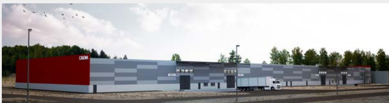
Volume Terminal, Katrineholm, under construction
